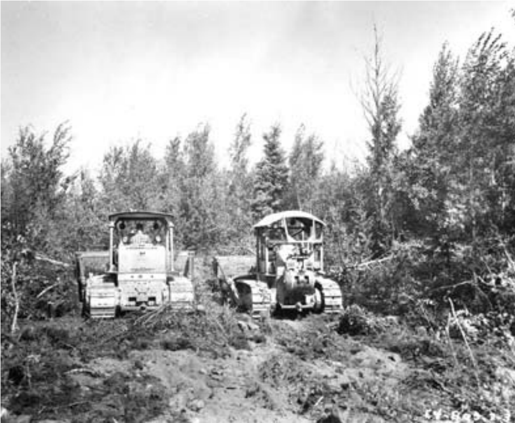
Construction on Hanson Lake Road, circa 1958.
