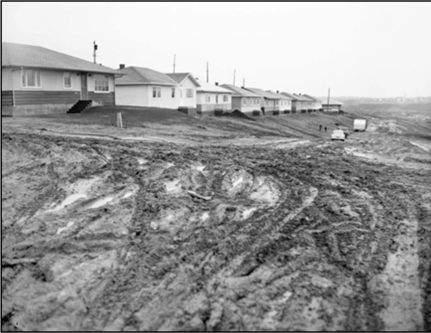
Impassable roads in a new subdivision, 1954.
