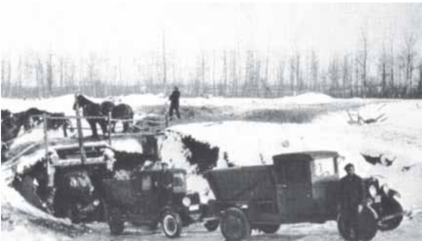
Road Construction, Elk Island National Park, 1930s
