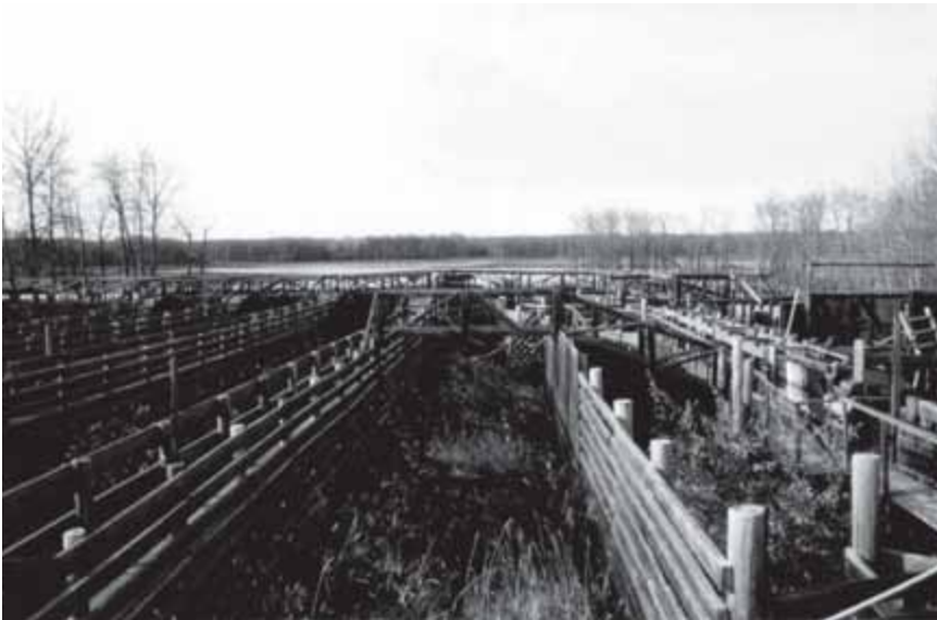
Bison processing facility, Elk Island National Park in 1992 These corrals were built in the 1930s to assist in rounding up bison for slaughter, for disease inspections, and for transporting to other centres.
