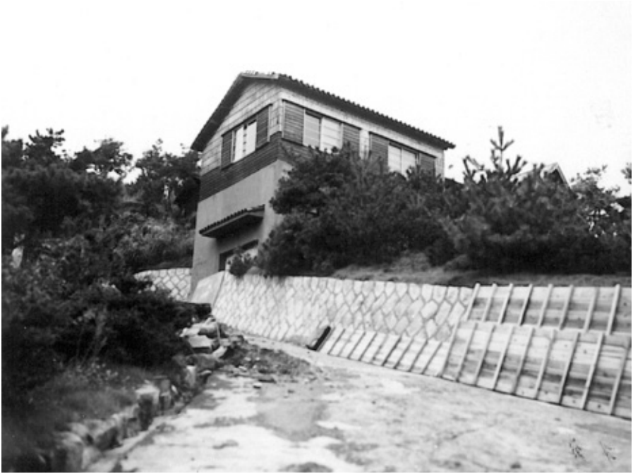
Ingelore's second home in Kobe with the prominent retaining wall.
